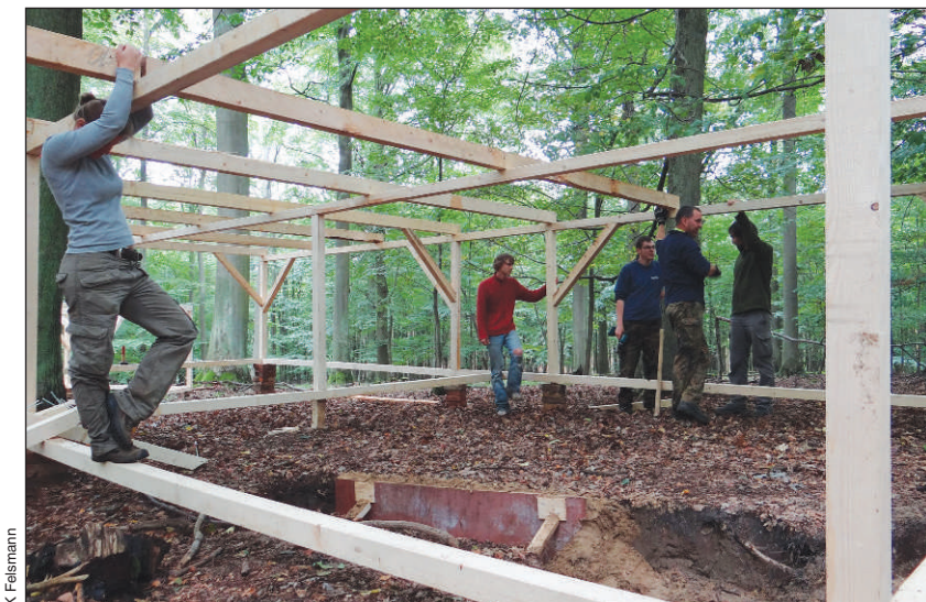
Figure 1. Construction of a series of roofs used at a rainfall reduction site. In the project, called BE-Dry, roofs were erected in forests in Germany to manipulate soil water levels. The interactions between plant and microbial diversity, and subsequent feedbacks to soil physical and hydrological properties, were observed over the growing season.
